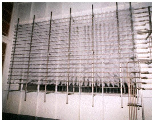
**Figure 2. High pressure fogging manifold system installed in the duct of a heavy-duty gas turbine. All stainless steel (316L) construction is used. Induced pressure drop is exceedingly small and not measurable.**
