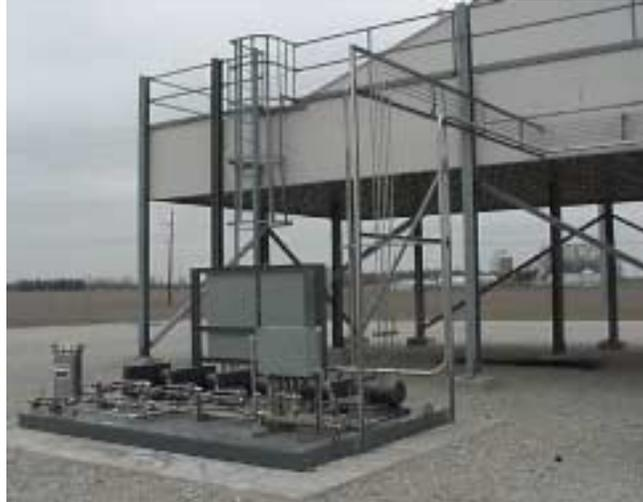
**Figure 1. Typical high pressure fogging skid. The feed lines from the high pressure pumps to the inlet system can be seen here. Retrofit installations can be accomplished in 2 days on most gas turbines.**
